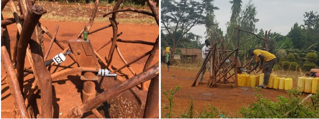
Figure A11.7. Borehole 1 near Jinja.
