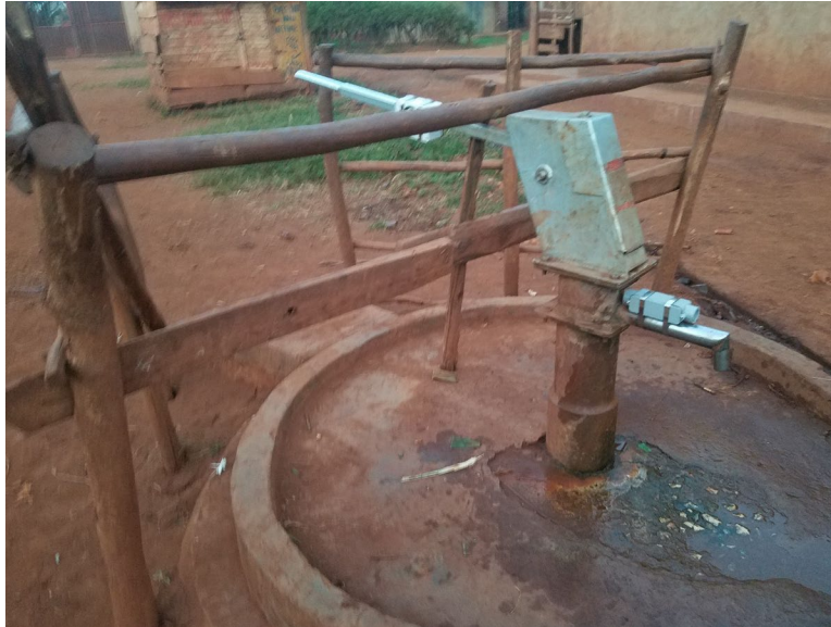
Figure A11.11. Borehole 2 near Jinja.
