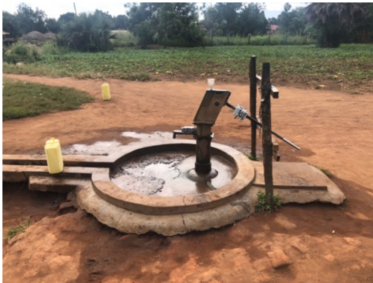
Figure A11.12. Borehole 3 in Gulu.
